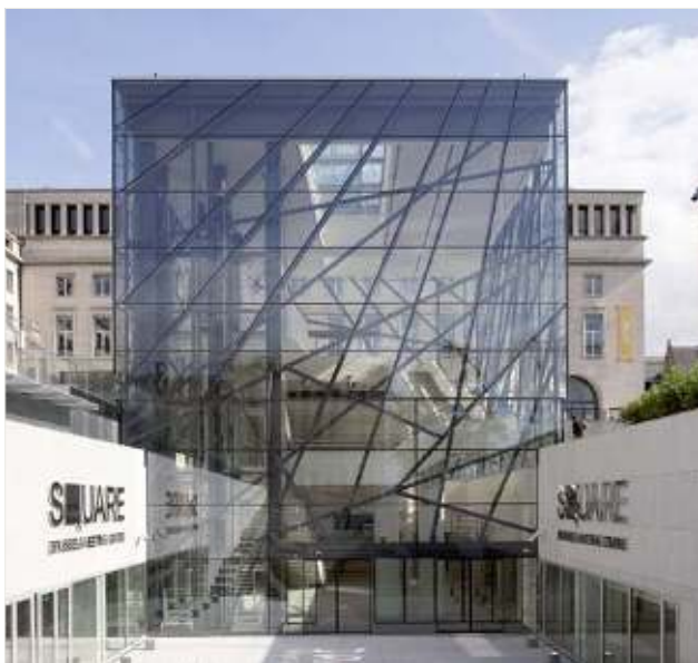
The new congress palace in Brussels, opened in September 2009. The sheets for the architecturally fascinating 14 metre high glass cube in front of the main entrance were supplied by LEROBEL. Each of the Sanco plus® laminated sheets has its own size and shape. Not a single sheet is rectangular!
